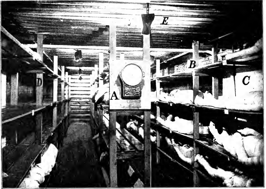
FIG. 181.—Refrigerating room. A , recording thermometer and middle tier of shelving; B and D , tiers of shelving; C , brine tank; E , pipes of refrigeration apparatus.
